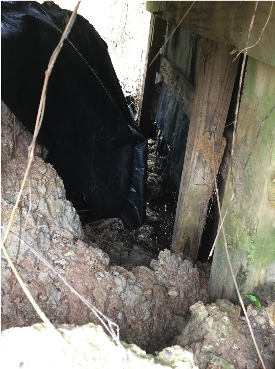
Figure 6. Levee erosion on the left side (looking downstream from the wetland to the pond) of the weir spill way
