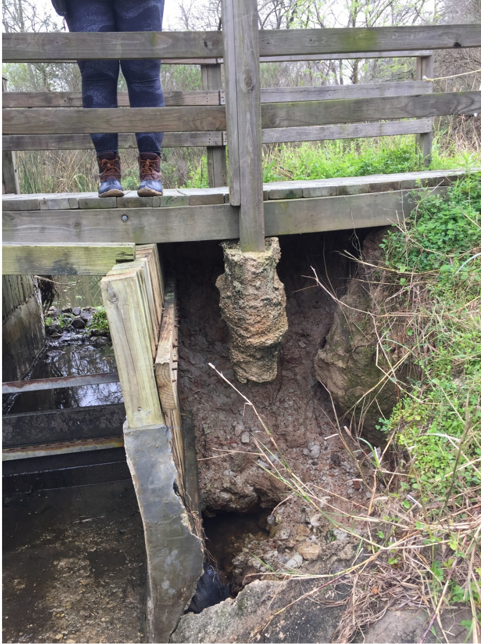
Figure 5. Erosion of levee around the spillway weir. Facing upstream from pond into primary wetland complex.
